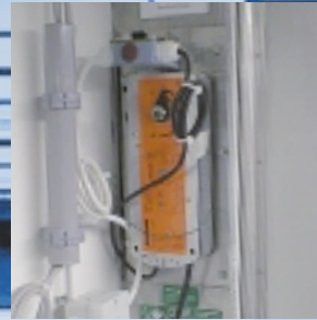
Motorized fire and smoke dampers protect both people and property
