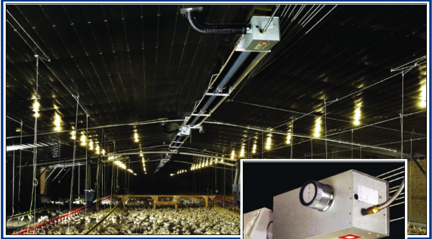
New Cold Air Stopper Option. Improves heating efficiency by preventing cold air during winter (warm air during summer) from entering your poultry house when the heating system is off.
