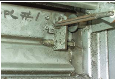
Fusible rod melts at 165°F.
