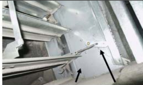
Negator spring Fusible Rod
